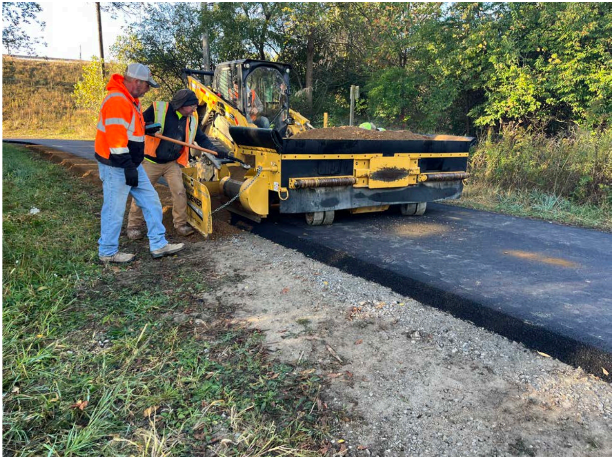
Lakeland Asphalt placing shoulder gravel on the Mike Levine Lakelands Trail.
