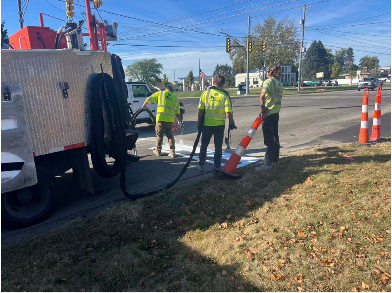
PK Contracting placing stop bars on Parnall Road.
