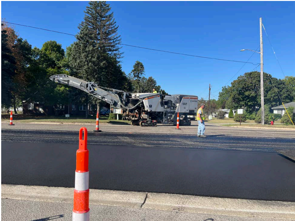
Lakeland Asphalt Cold Milling at Lansing Avenue and Parnall Road intersection.
