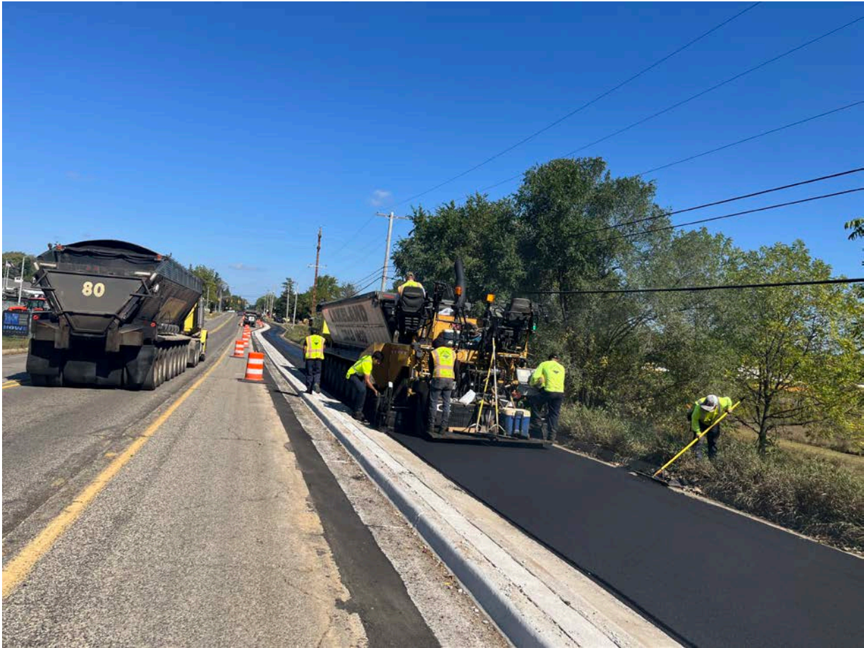
Top course paving on Lansing Avenue and Parnall Road.
