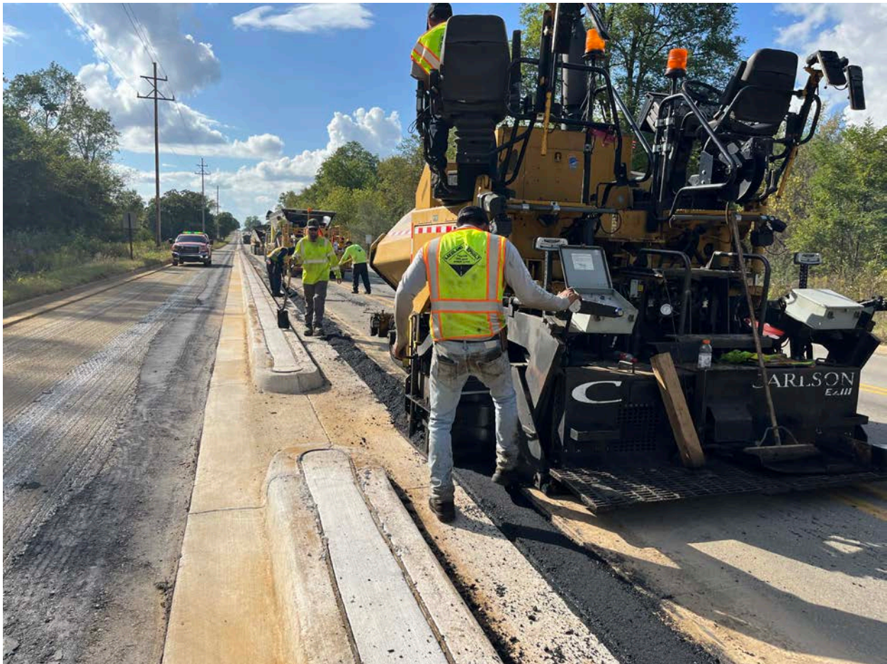
Hand patching placement on Lansing Avenue and Parnall Road.
