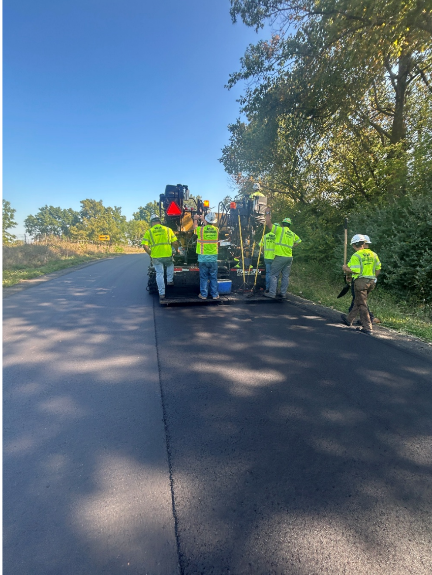
Top Course Paving on Moscow Road.
