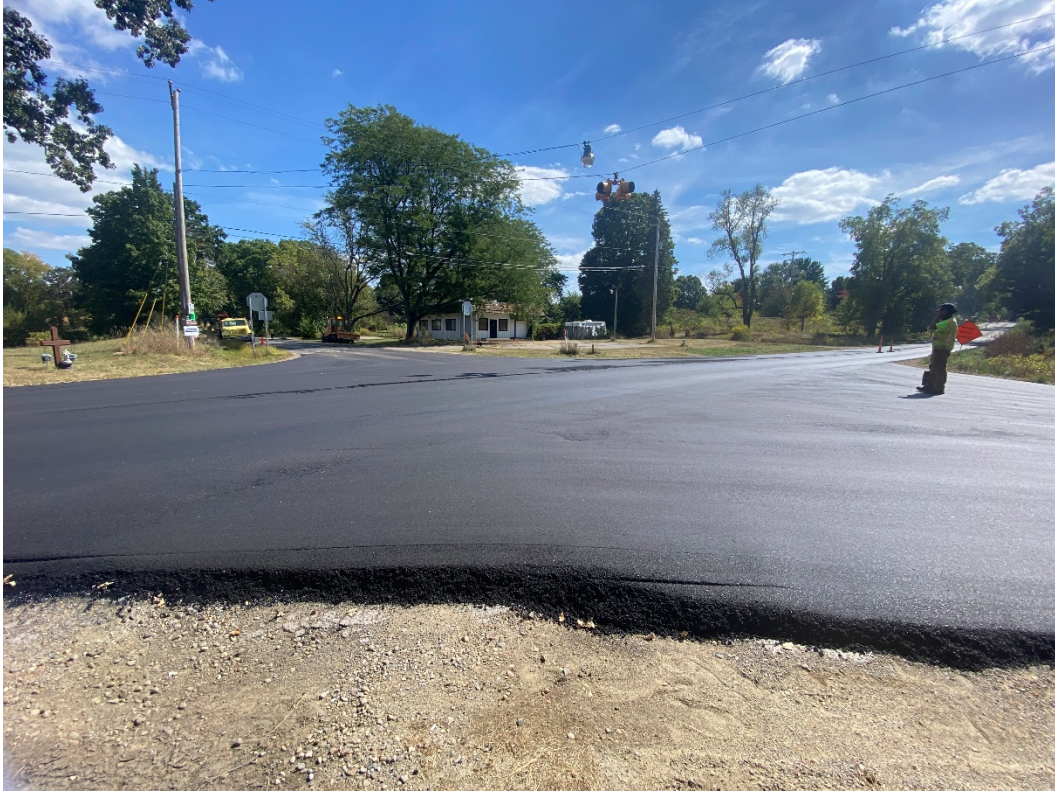
Wedge Course Paving Moscow Road and Hanover Road intersection.
