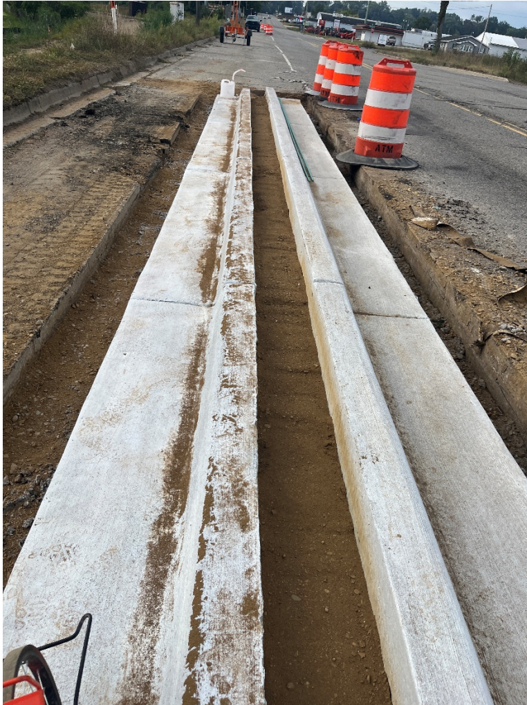
Compaction and aggregate placement for center concrete median.
