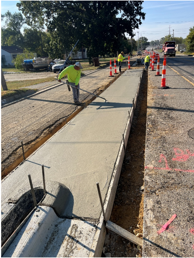
Concrete driveway placement on Lansing Avenue.
