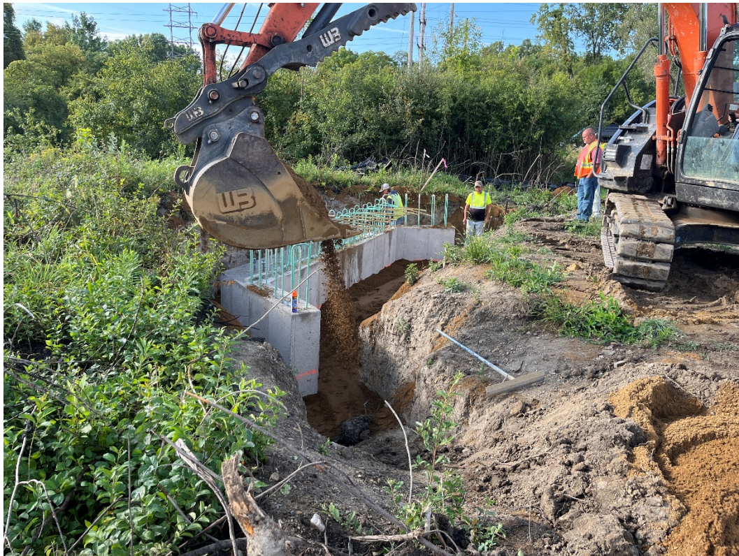
Backfilling material for the pedestrian bridge over the Grand River.
