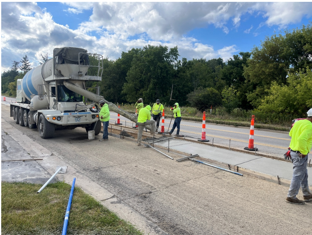
Concrete driveway placement on Parnall Road.
