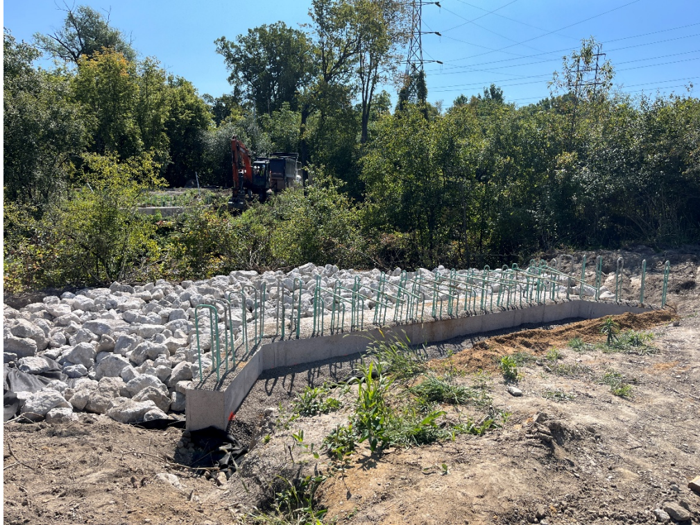
Rip Rap at the pedestrian bridge over the Grand River.
