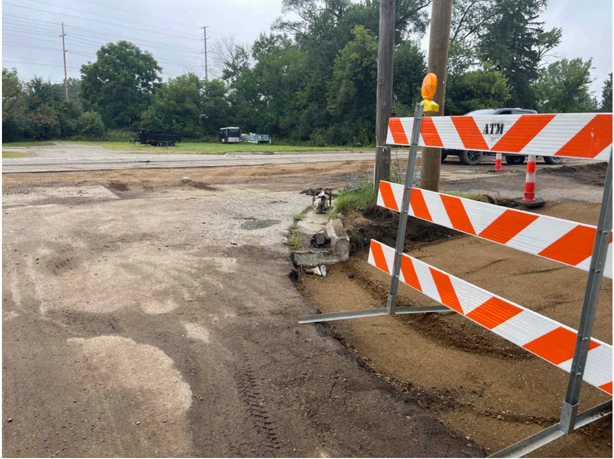
L.J. Construction Shared-Use Path preparation
