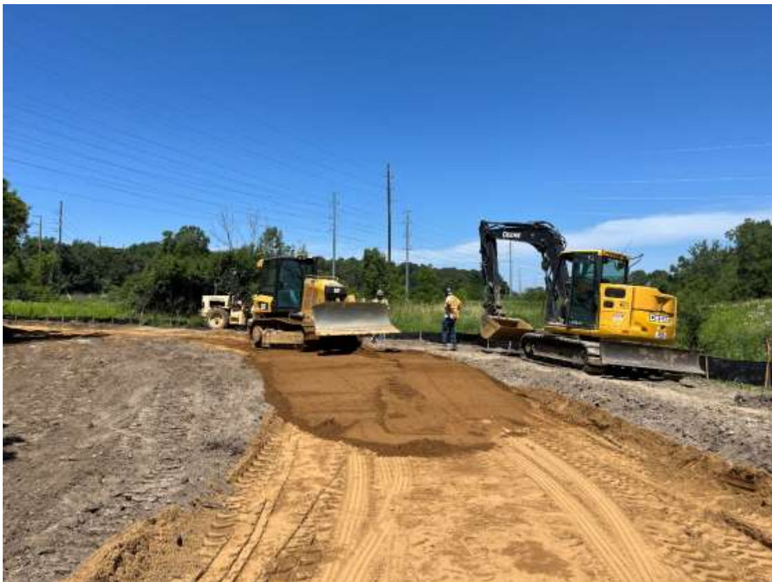
Pedestrian Bridge Concrete Abutments
