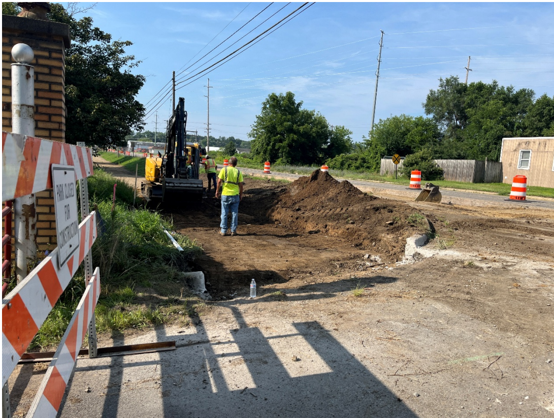
Parnall Road Aggregate Base Grading
