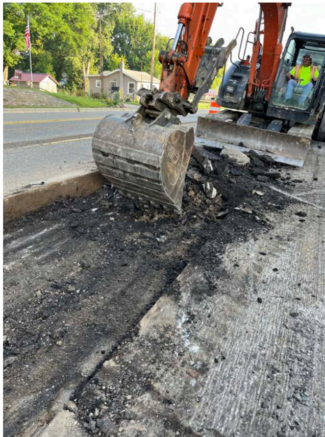
Lansing Avenue HMA Surface Removal
