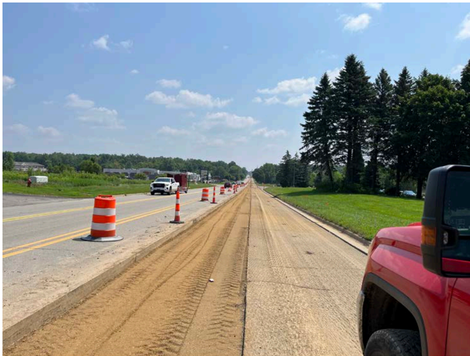
Parnall Road Aggregate Base placement
