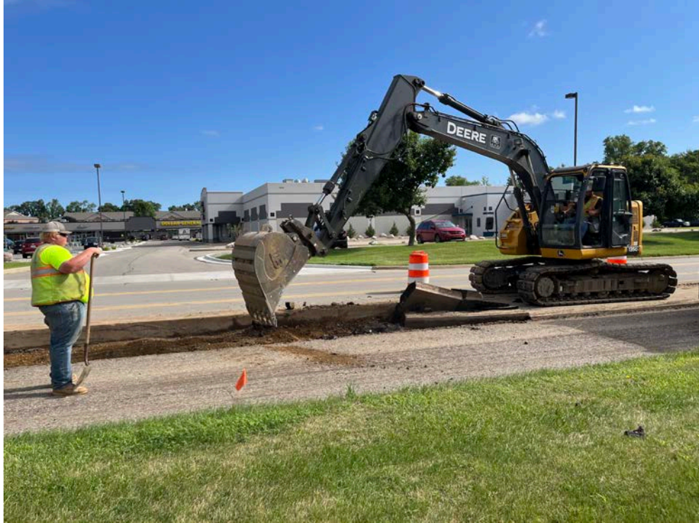
Parnall Road HMA Surface Removals
